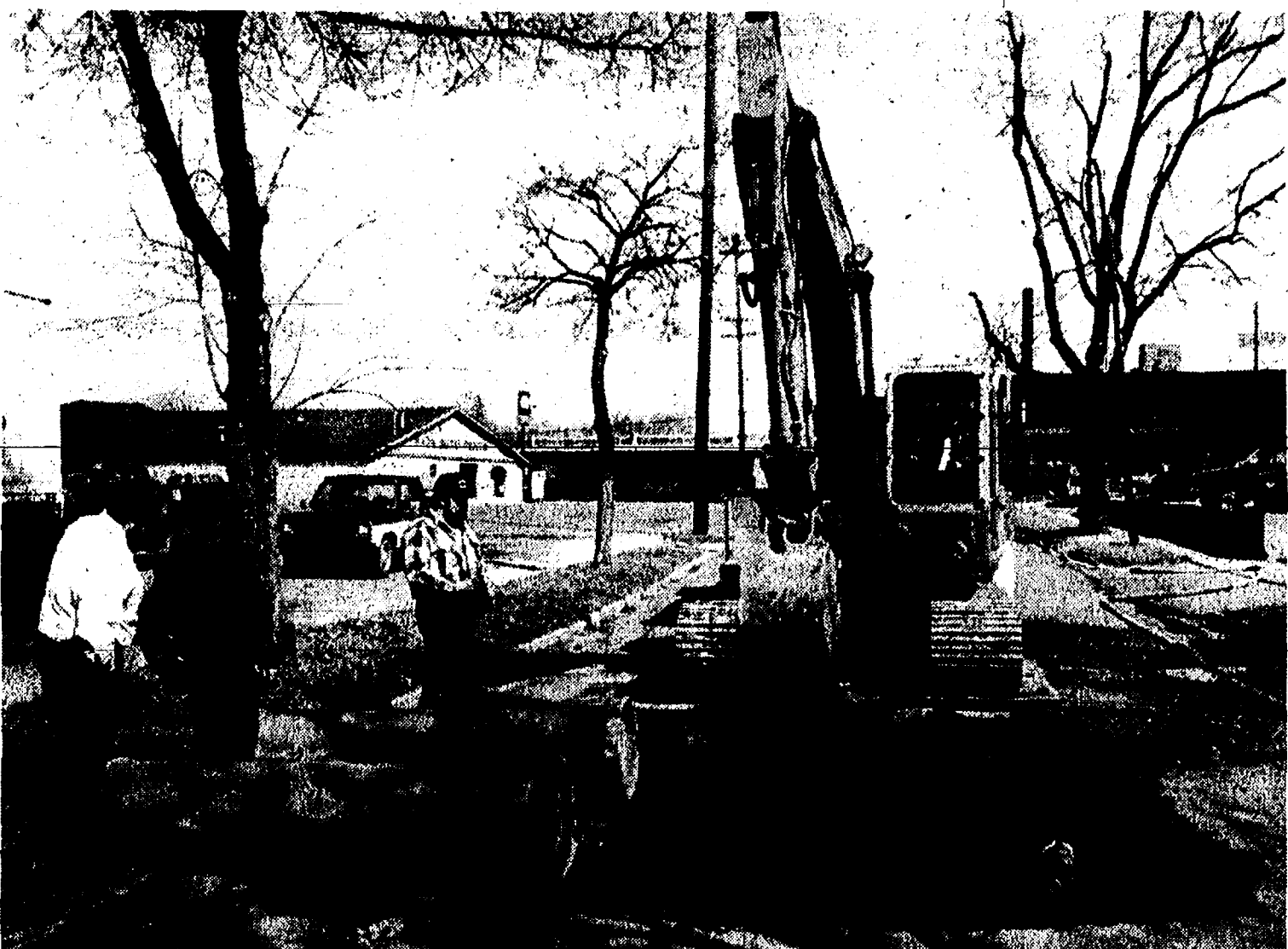
SEWER LINE is being replaced in several areas of town as part of an effort to upgrade the capacity of the new wastewater treatment plant. Here workers dig down to replace pipe on North St. Recent warm weather has made the job a little more pleasurable.
